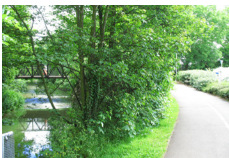
Existing conditions along Botany Stream edge
