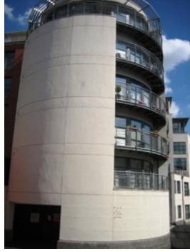
Car parking entrance discreetly accommodated into a corner building
