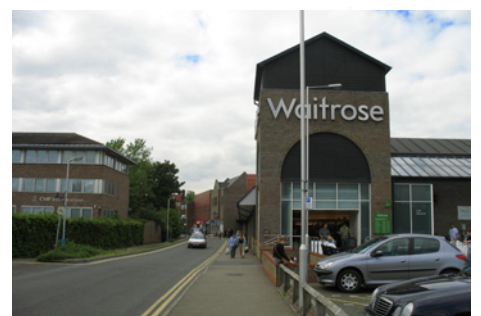
Sovereign Way needs reinforcing
